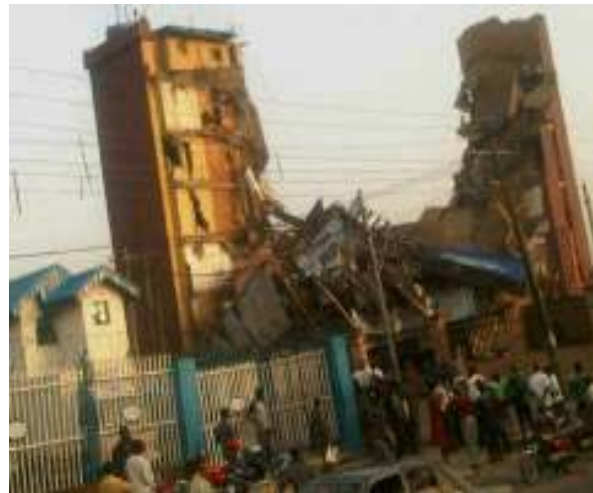
Picture of The Don de Dieu Plaza, a 6-storey building, which was located at 11, Aderibigbe Street, in Maryland, Lagos which collapsed on Wednesday, 26 th October, 2011
