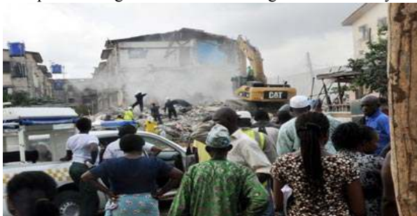
*Picture of a two storey building that collapsed at the end of Church Street Jakande Estate Extension, Oke-Afa, Isolo, Lagos State, on Wednesday 6 th November, 2013.
